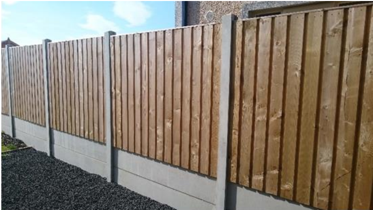
Concrete Post & Wooden Panel Fence
