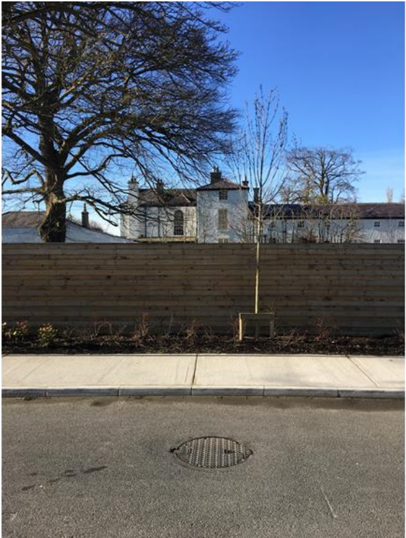
Double Sided Treated Wooden Panel Fence With internal concrete post & Gravel Board
