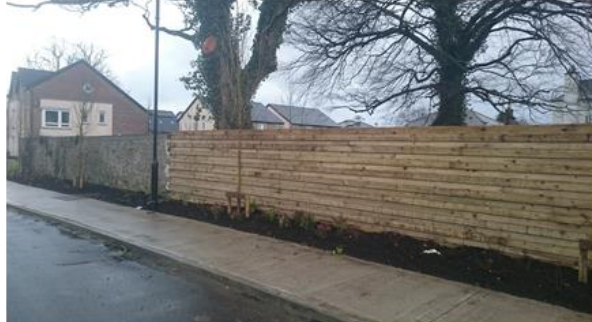
Double Sided Treated Wooden Panel Fence to Boundary & Existing Hedge
