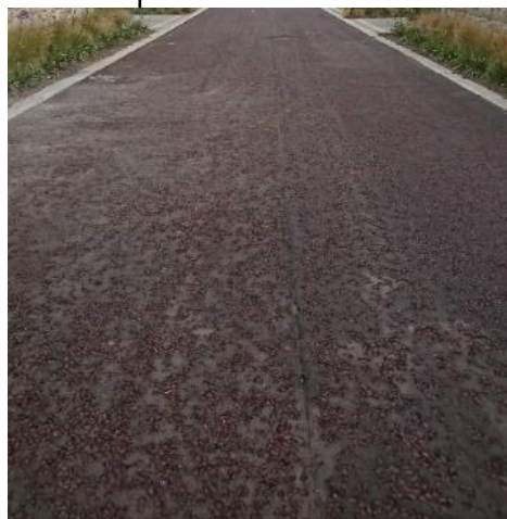
Shared surface material Tarmacadam Hot Rolled with Red- Coated Chippings
